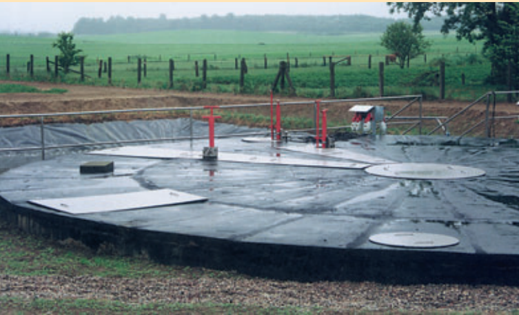
mounting Turbo-Jet in a covered basin (refitted small water clarification plants) only mounting visible manual dismantling without emptying the basin
